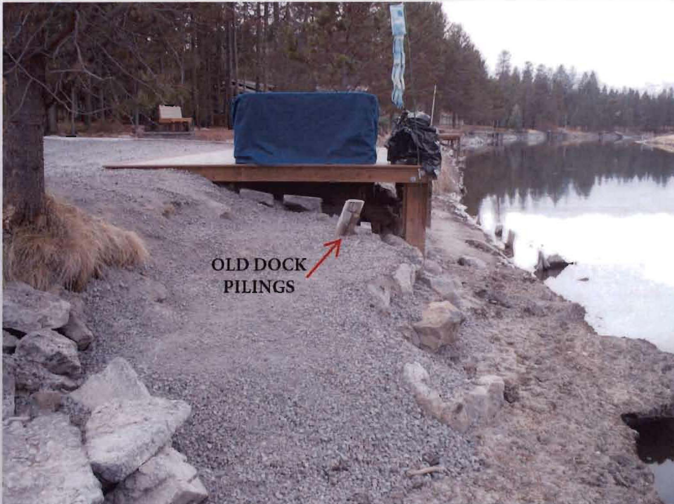
Completed over-water dock and over-land platform for access to the dock on northern edge of property, looking west down the Deschutes River. Photo taken Winter of 2009.
