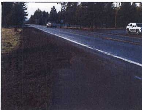
Exhibit 3: Vehicle overtracking in SW corner
