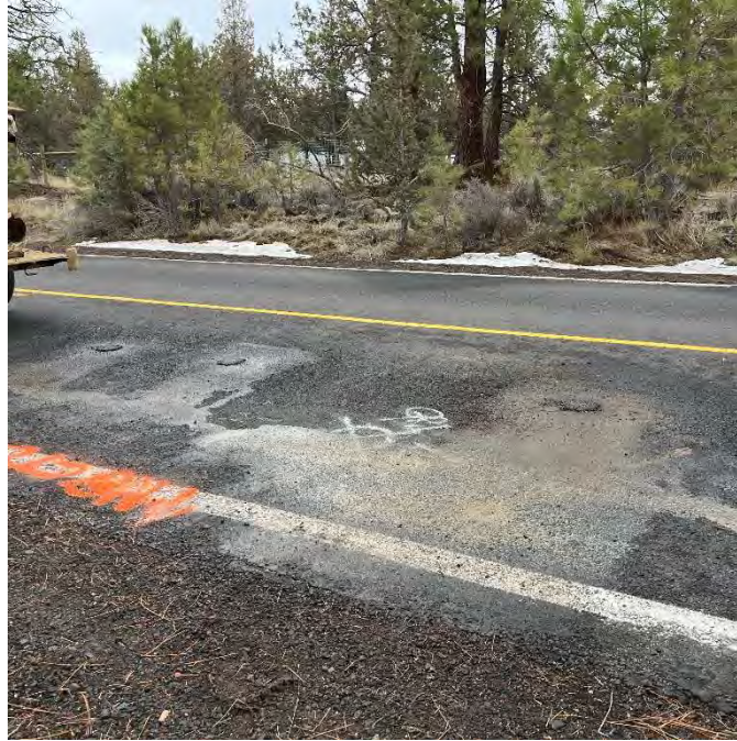
a. Boring PB-1 Location
