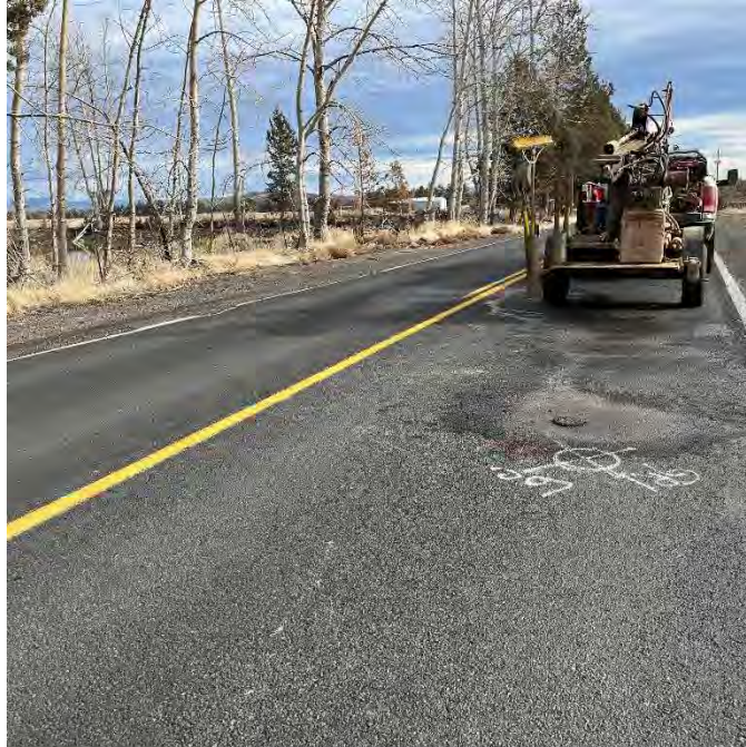
a. Boring PB-4 Location
