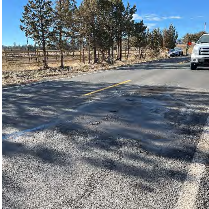
a. Boring PB-5 Location
