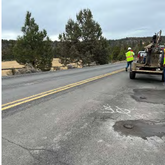
a. Boring PB-12 Location
