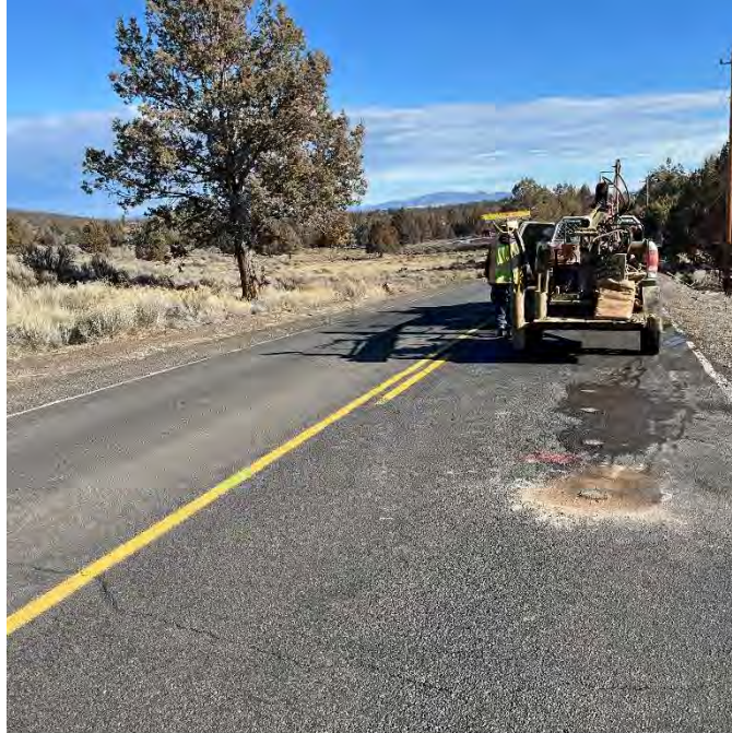
a. Boring PB-6 Location
