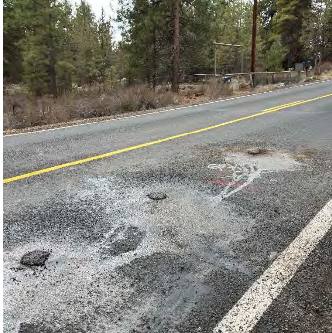
a. Boring PB-3 Location
