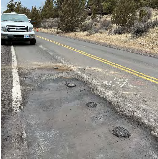
a. Boring PB-10 Location
