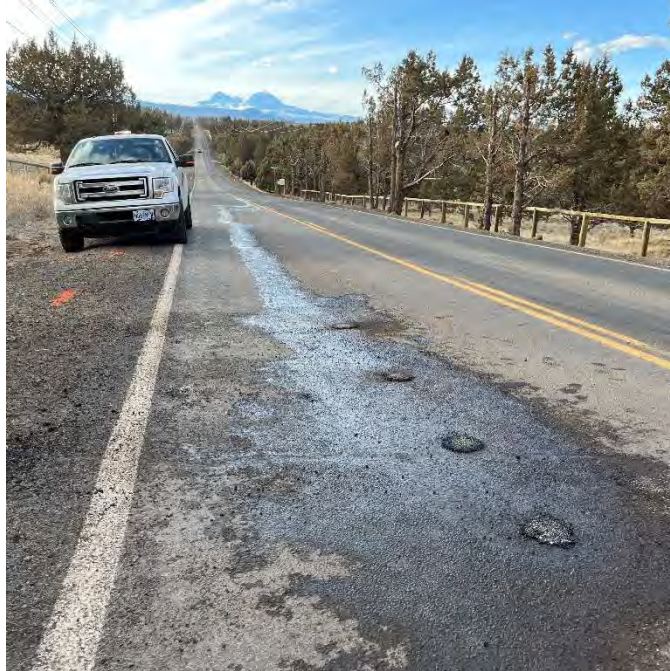
a. Boring PB-8 Location
