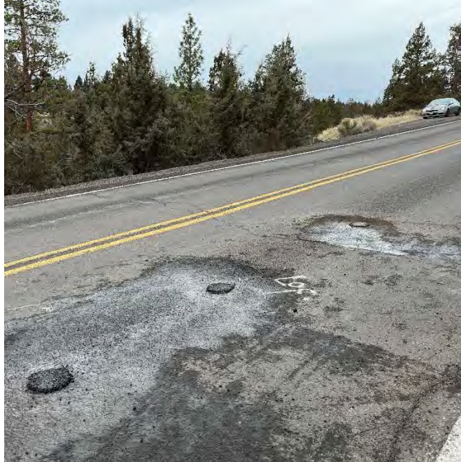
a. Boring PB-11 Location
