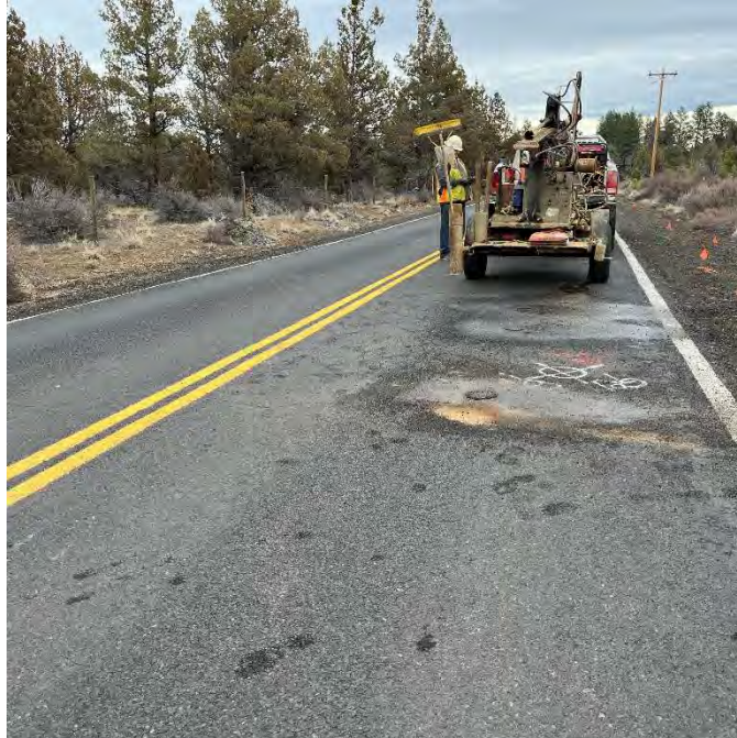
a. Boring PB-2 Location
