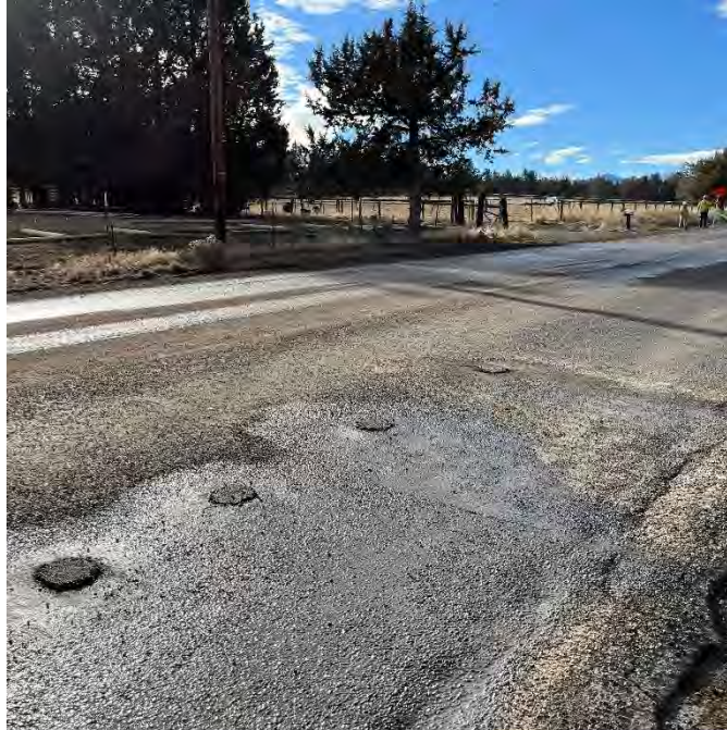
a. Boring PB-7 Location
