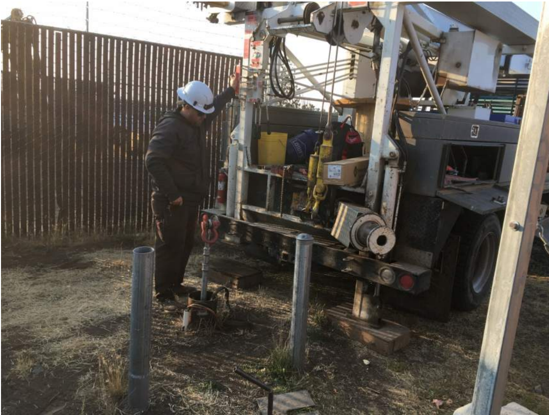
Thompson Pump and Irrigation staff removing the existing pump.
